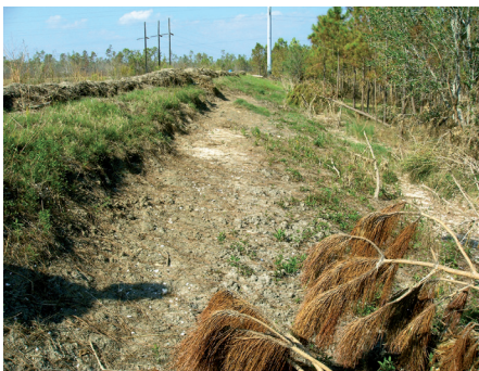
Figure 10 Erosion by waves and trash on the crest.
