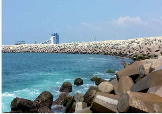
Figure 22 A rubble mound structure with corelocs. Very efficient in dissipation of wave energy.
