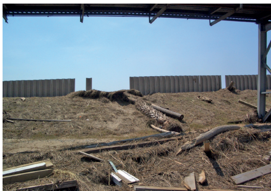
Figure 12 Breaking of pvc-sheet piles by hammering logs.
