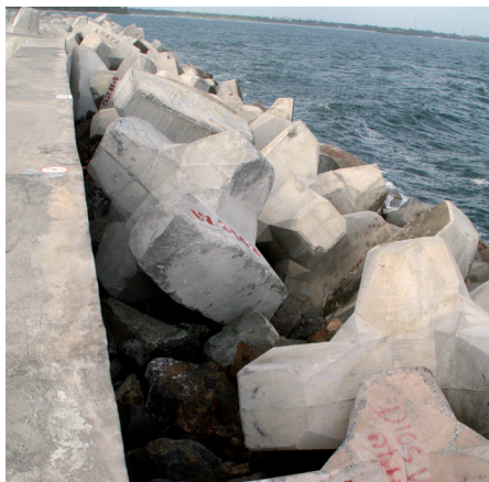
Figure 4 A gap at the crest appears after the first storm, if settlement has not occurred during construction.
