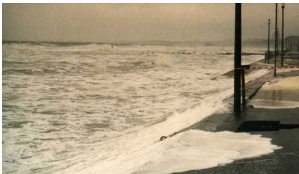
Figure 1. Wave overtopping on a revetment seawall
