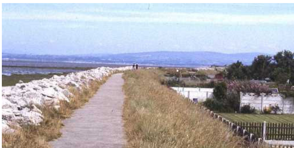
Figure 6. Defended area below seawall and foreshore (saltmarsh) level
