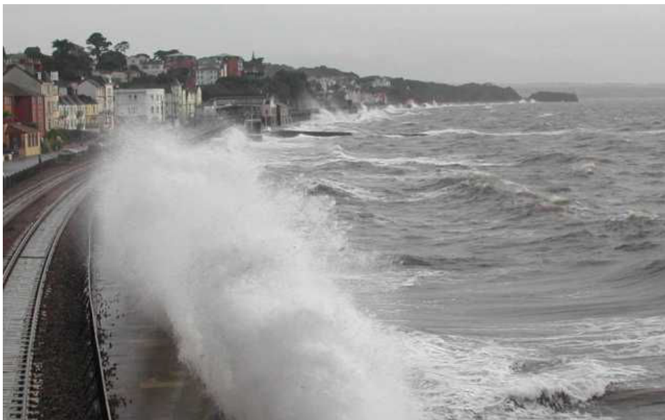
Figure 3. Wave overtopping on a battered / vertical seawall
