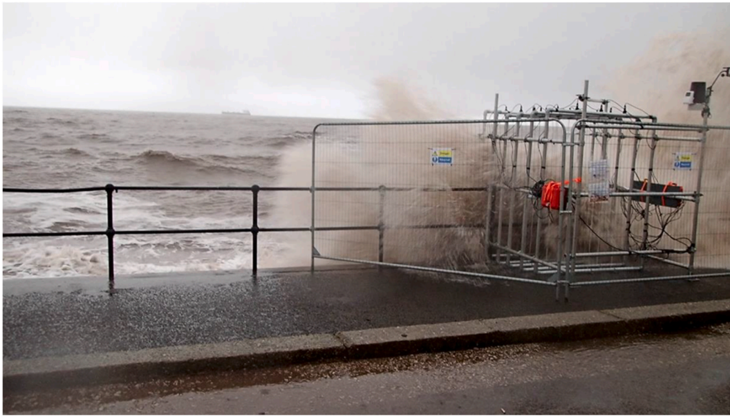
Fig. 4. WireWall system installed at Crosby as a wave overtops the structure.
