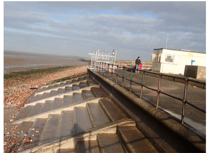
Fig. 2. Photo of the coastal defence at Crosby with foreshore exposed at low tide.
