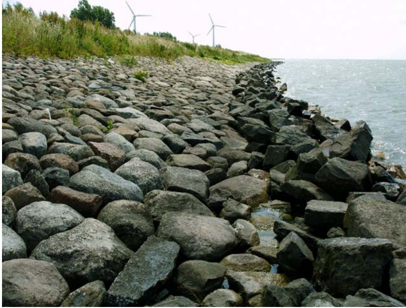
Figure 2. Pitched rock slope along large lake with a randomly dumped rock berm in front
