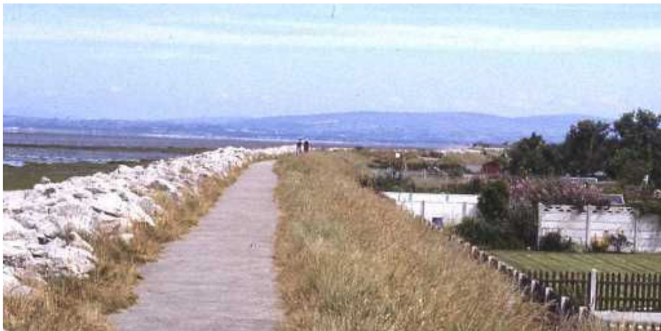
Figure 4: Defended area below seawall and foreshore level
