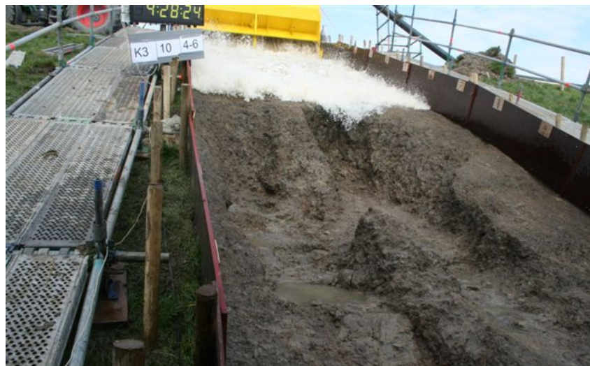
Figure 8: Wave overtopping test on bare clay; result after 6 hours with 10 l/s per m width
