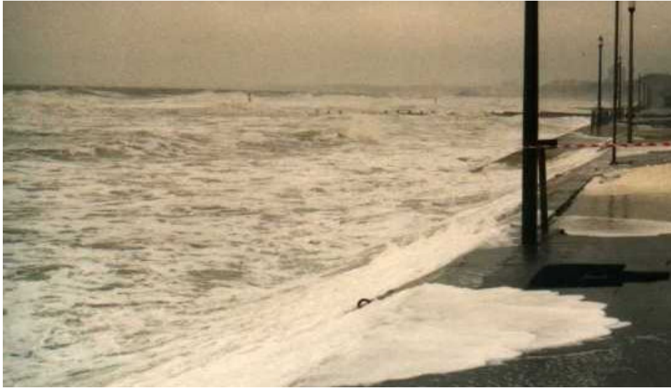
Figure 1: Wave overtopping on a revetment seawall
