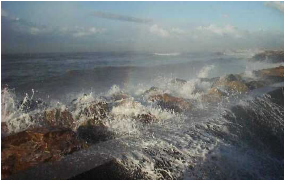
Figure 3: Wave overtopping on a rubble mound breakwater (courtesy Prof. Leo Franco)
