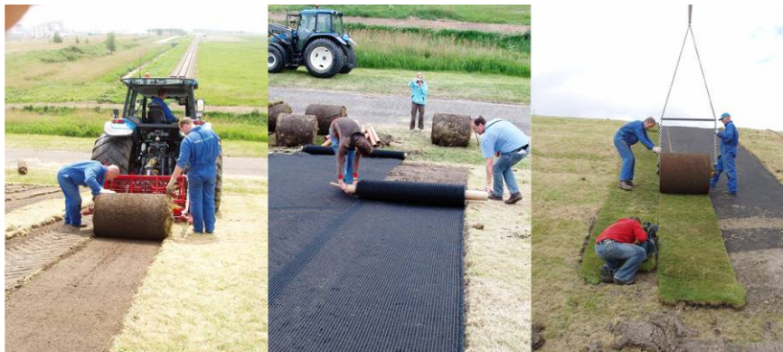
Figure 4: Illustration of obtaining the SGR: cutting of grass (left), placement of geosynthetic (middle) and unwinding of the big rolls (right)
