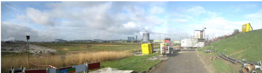
Figure 6: Wide angle view of test set-up at the inner slope of the Groningen sea dike
