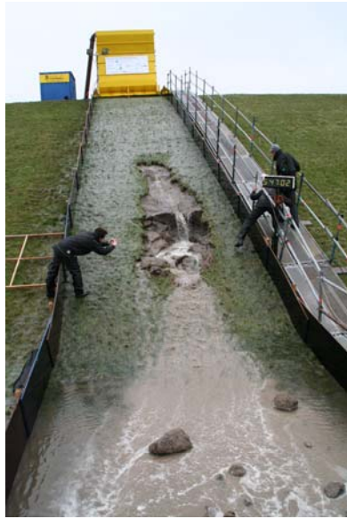
Figure 9. Erosion at inner slope for 75 l/s per overtopping
