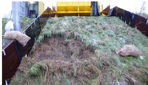
Figure 5. End result of section 3.
