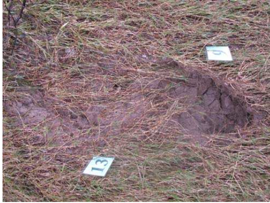
Figure 5. First damage on a Bermuda grass slope, section TL_03.
