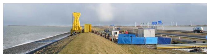
Figure 13. Set-up of the Wave Overtopping Simulator close to a highway.
