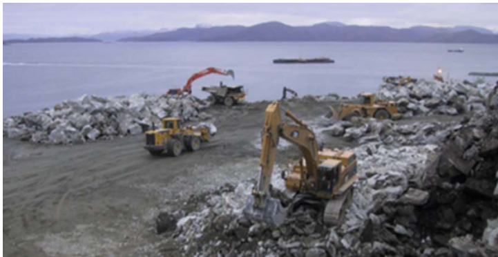
Figure 4. Sorting of material from the blasting pile with excavators and front loaders, loading of truck from the stock pile. The Hammerfest project.
