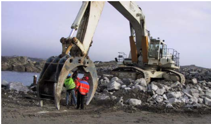
Figure 6. A 110 t excavator with a rock prong, Sirevåg breakwater.
