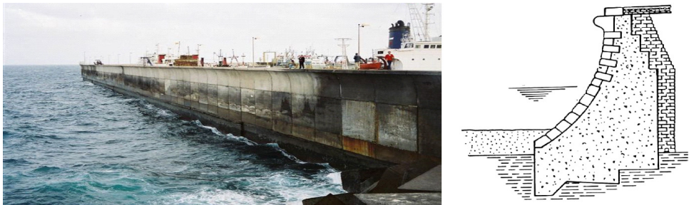
Fig. 16.17. An example of a modern, large vertical breakwater with wave return wall (left) and cross-section of an older seawall with recurve (right).
