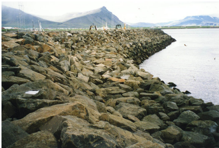
Fig. 15.15. Icelandic berm breakwater.
