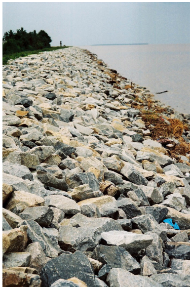
Fig. 15.1. 1:4 rock-armored embankment.
