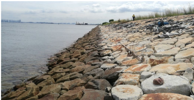
Figure 1. A typical pitched rock slope in Singapore.
