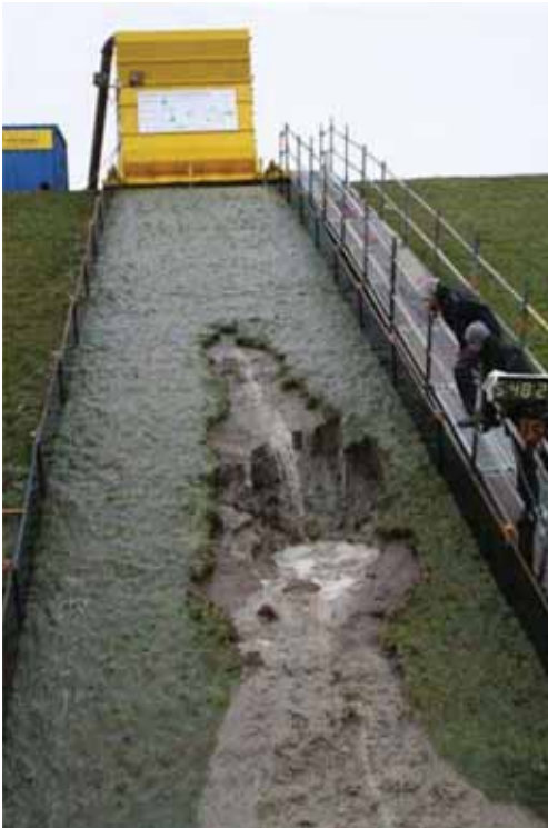
Figure 4. Damage to a dike section during a test with 75 l/s per m wave overtopping.
