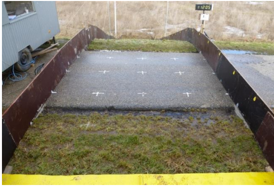
Figure 3. Revetment transitions from grass to asphalt and from asphalt to grass
