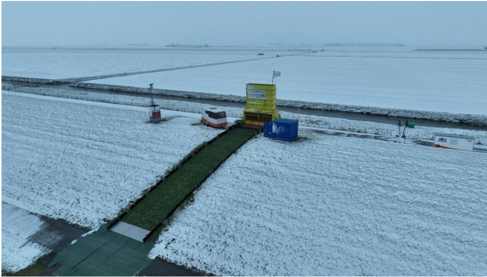
Figure 1. Wave overtopping tests on a real dike in the Carel Coenraadpolder in 2023. The yellow wave overtopping simulator (WOS) is placed on top of the dike crest facing the slope.
