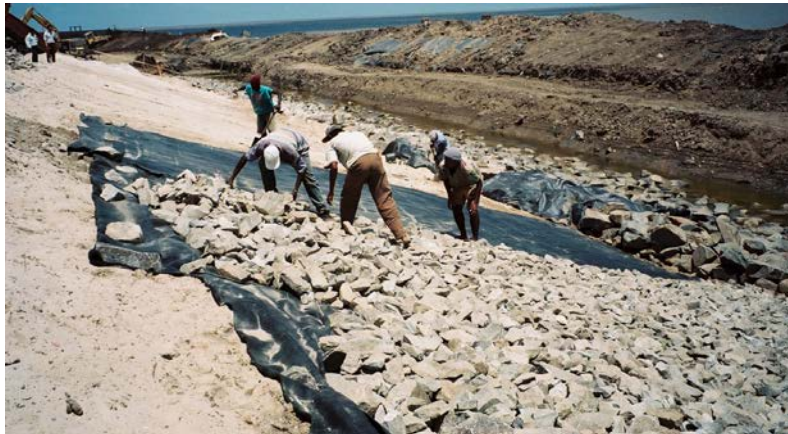
Figure 1: Laying small underlayer stones on a geotextile on sand.
