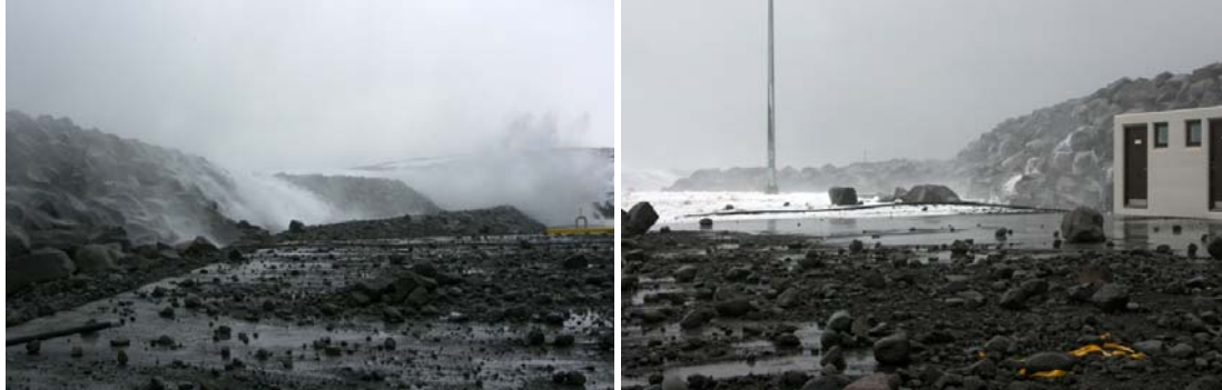
Figure 16. Husavik berm breakwater at the end of the 25 October 2008 storm. Gravel and small rock from unpaved area behind the crest washed upon the quay area.
